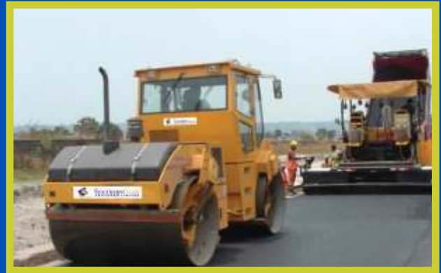
(Port Harcourt Project) Road Construction by Southernglow Ventures Limited.
