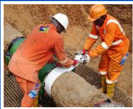
Cold cutting and Welding work on 24inches Oben-Ajaokuta Gas line for Nigeria Gas company
