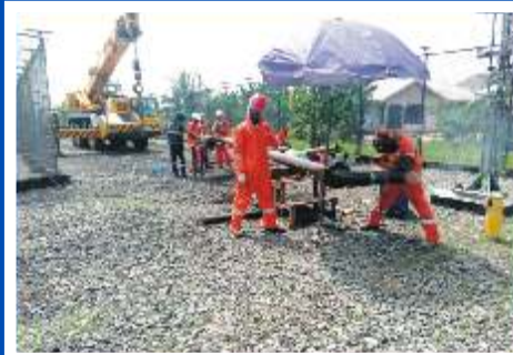
Manifold Upgrade Works
