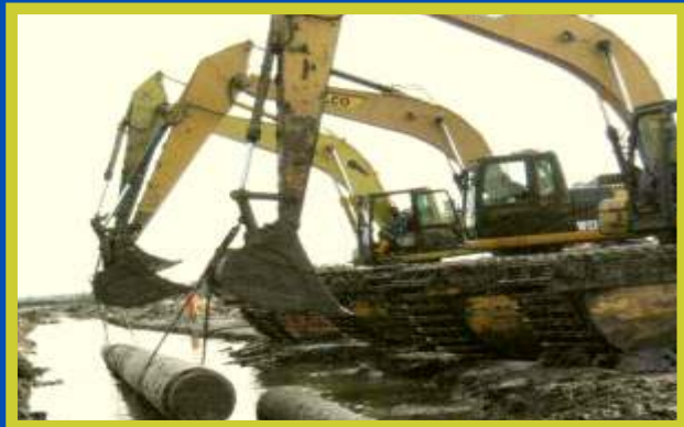
Pipeline Installation
