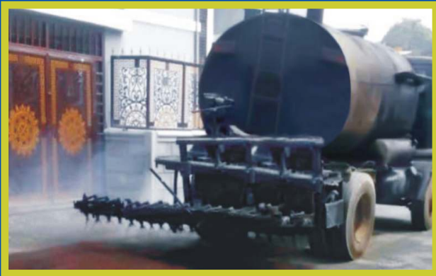
Road construction at Rumuibekwe Housing Estate, Port Harcourt.
